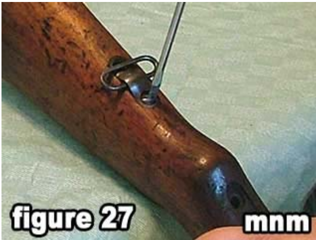
27) Loosen the front swivel screw .
